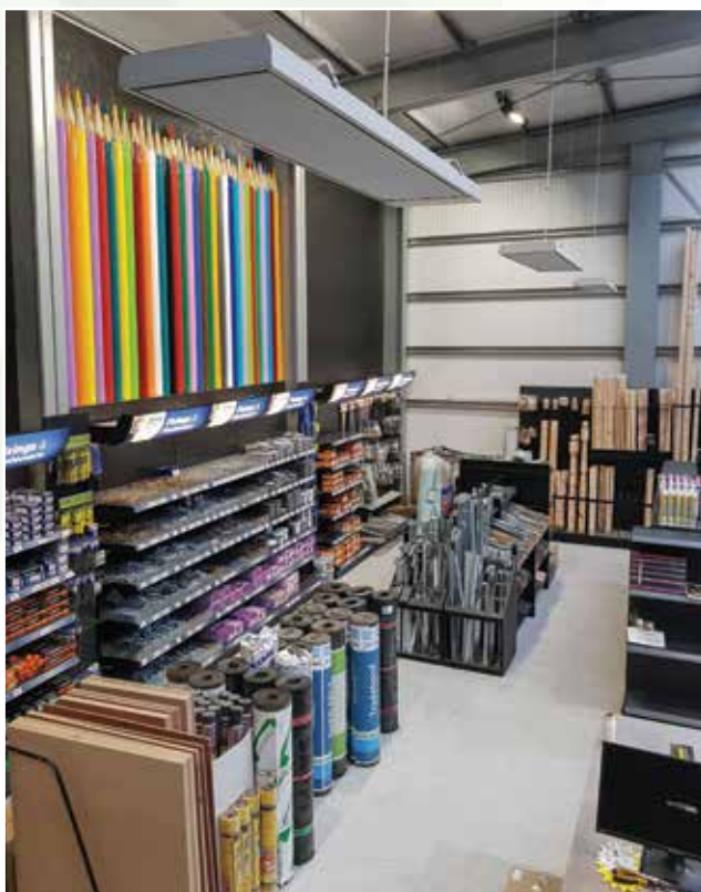
Radiant cassettes installed in a timber showroom in Bedford
